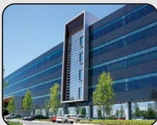
Panduit Corp. Worldwide Headquarters Tinley Park, Illinois 60487
